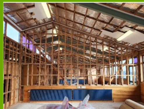
Main Block Stripped Out prior to reconfiguration.
