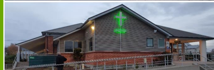
The recently completed re-clad project at St Mary's Milton.
